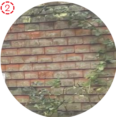
Clay wall tiles to match existing
