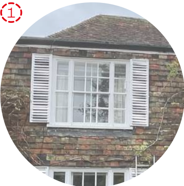
New timber sash windows to match existing
