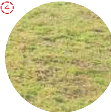
Sedum roof over single storey extension
