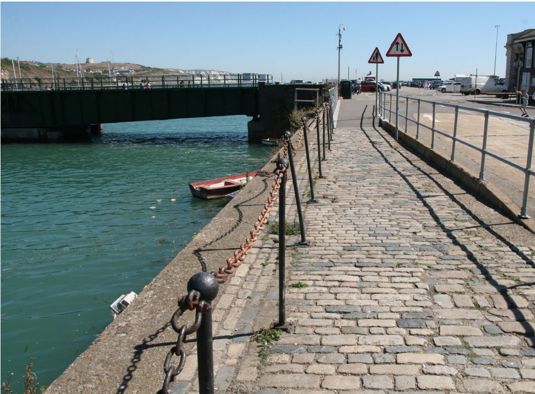
6. View along north edge of the Harbour, looking towards the Viaduct
