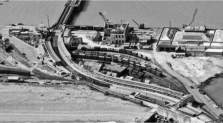
Fig 6.5.2 Folkestone Harbour Station
