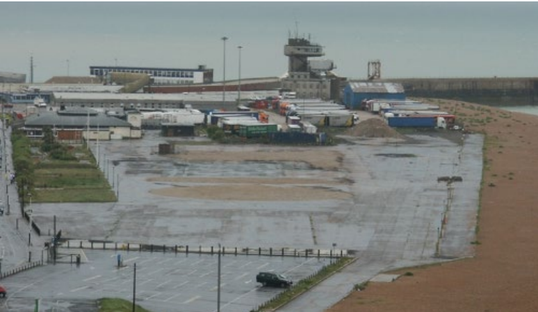
Fig 6.7.1 The Lorry Park & Concrete Beach
