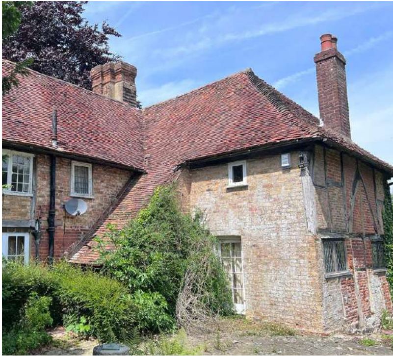
View of side / south-east elevation
