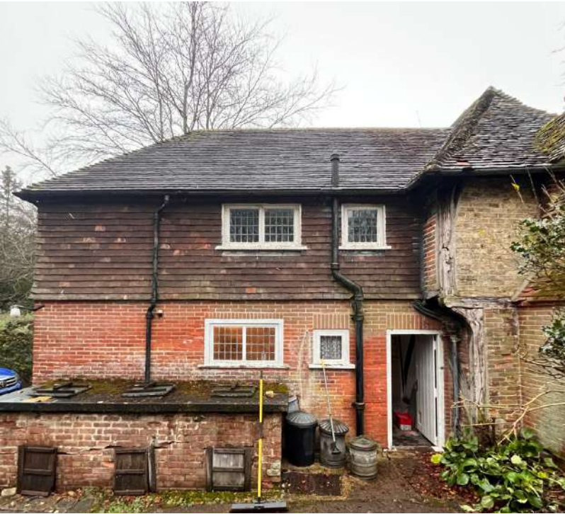
View of rear / south-west elevation
