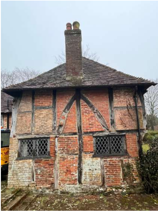
View of side / south-east elevation
