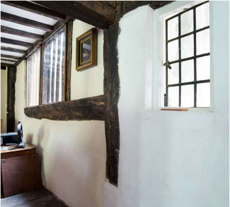
The Old School House: Finished interior
