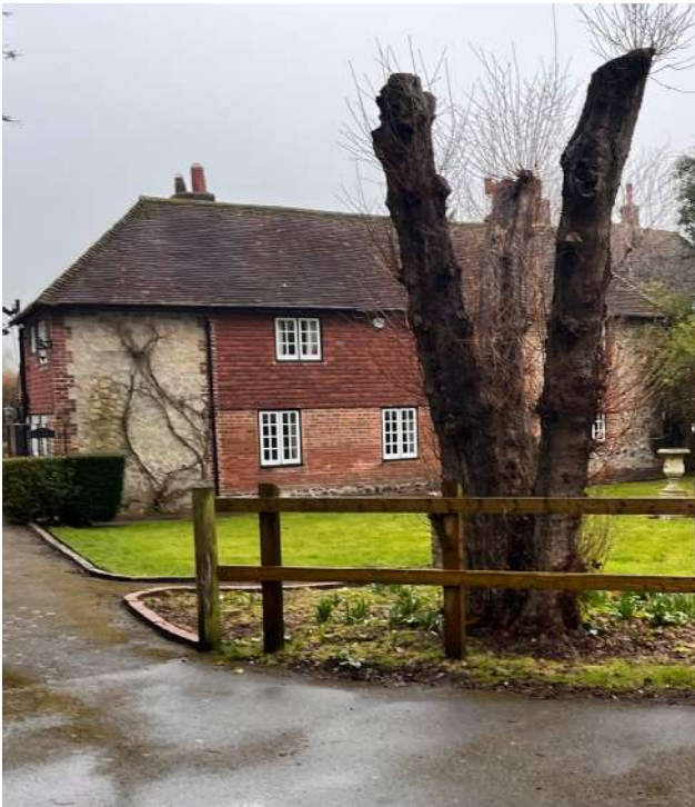
View of Ridge Cottage
