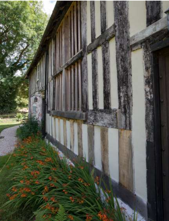
The Old School House: Finished exterior
