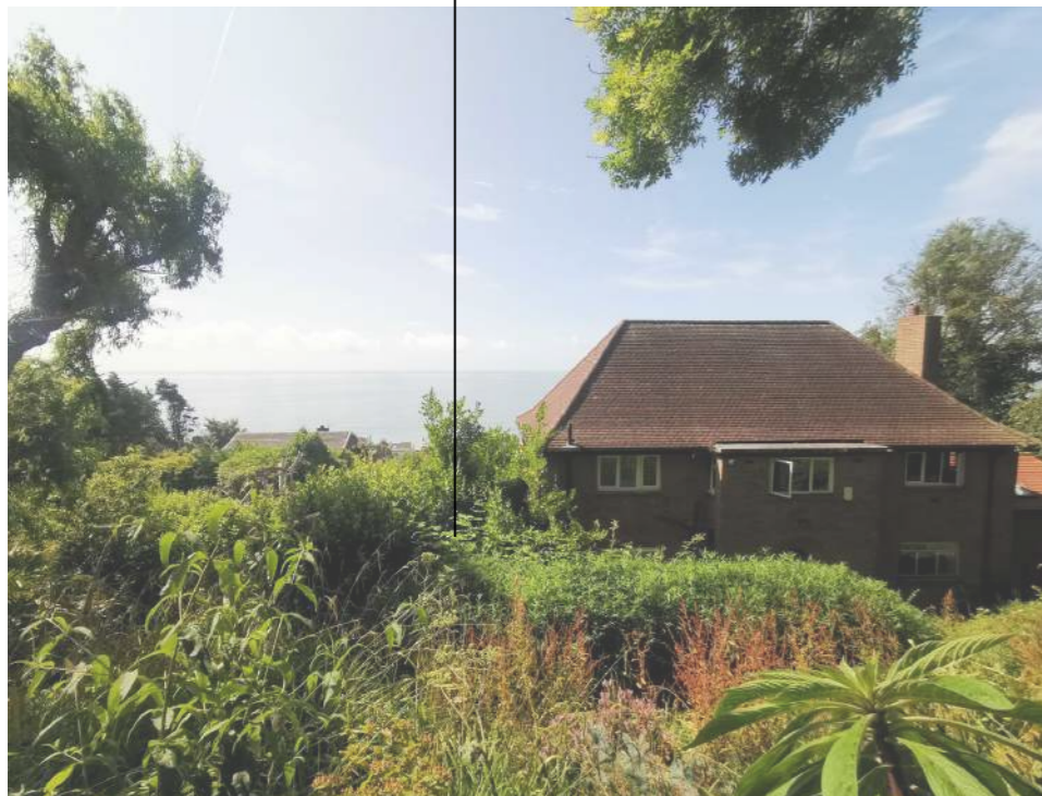
View D: view towards the rear facade of the building
