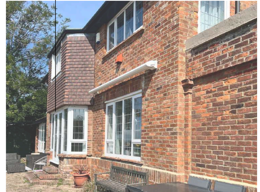
View C: view showing the front facade of the building
