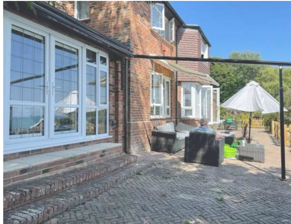
View G: view showing existing terrace
