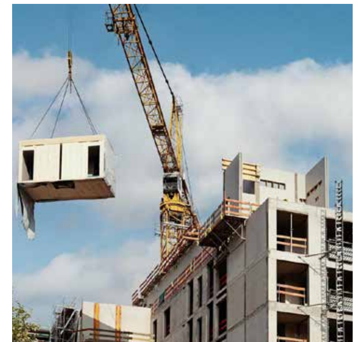
Units constructed offsite and craned into place
