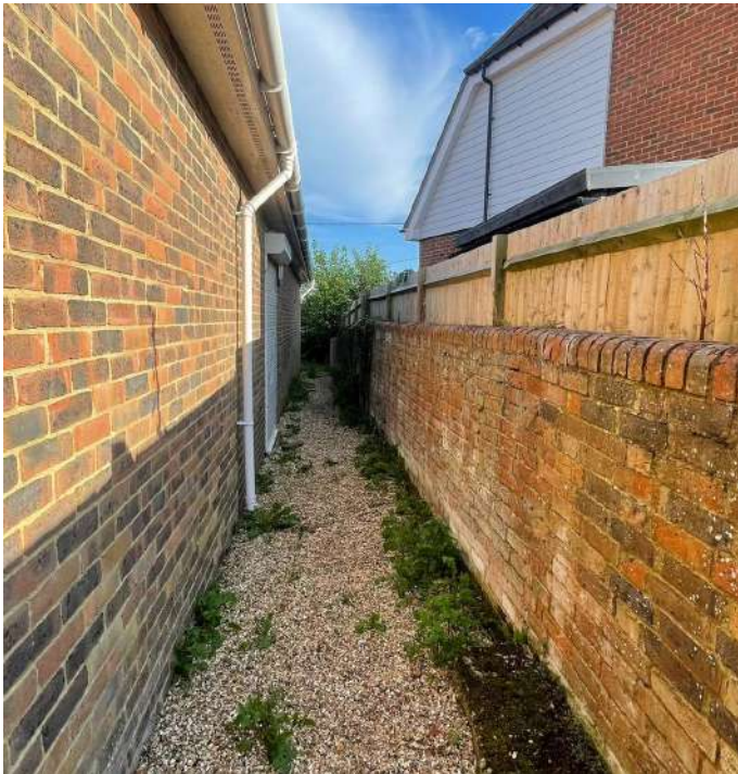
View of rear passage
