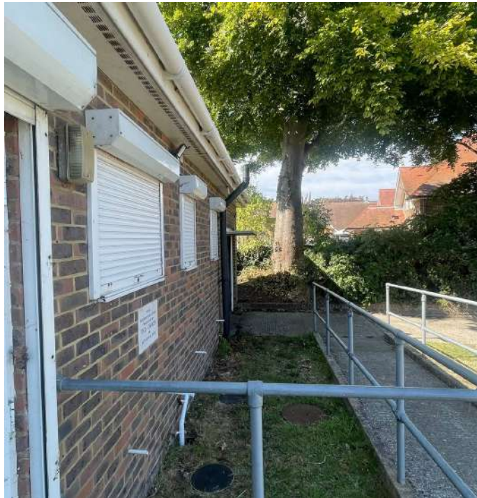
View of the existing access ramp
