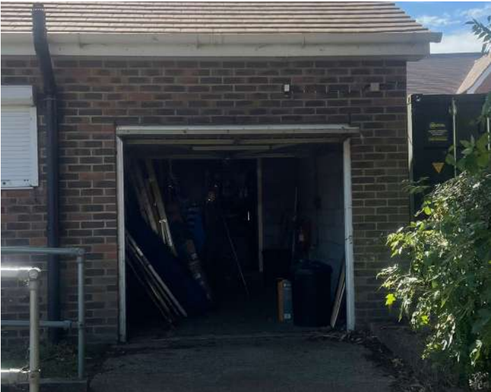
View of the existing garage door
