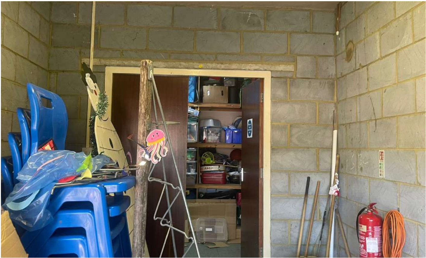
View of existing garage
