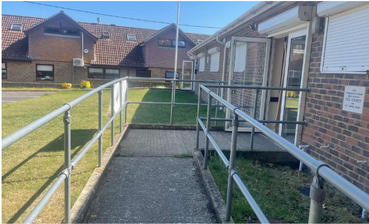
View of the existing access ramp and entrance
