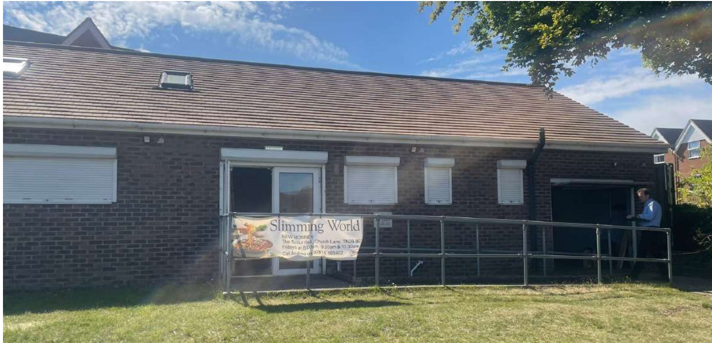
View of the main entrance, ramped approach and garage door
