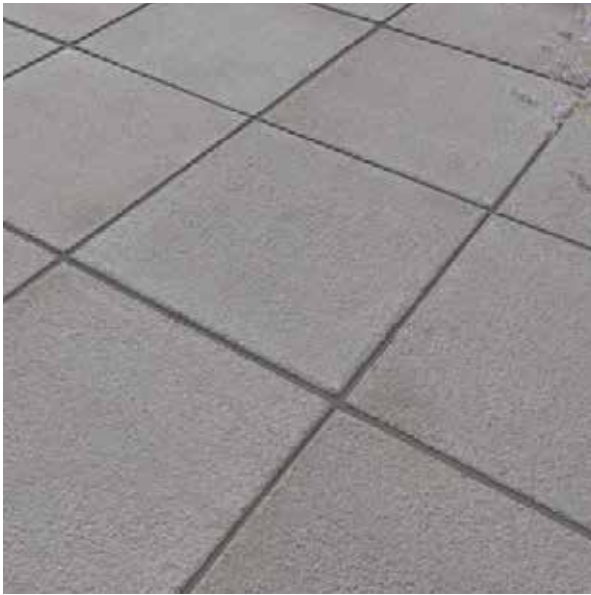
External Areas - Concrete Paving
