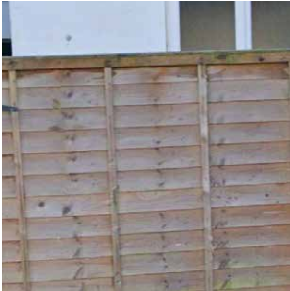
Boundary Fencing - Timber Panelling
