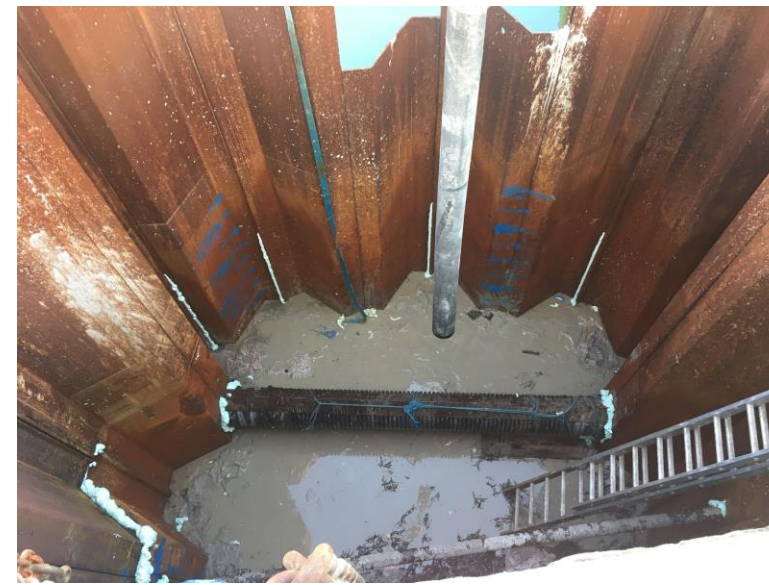
Figure 29 – Sheetpile closure sealed ready for underwater concrete.
