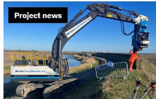
Figure 24b. Excavator and Movax
