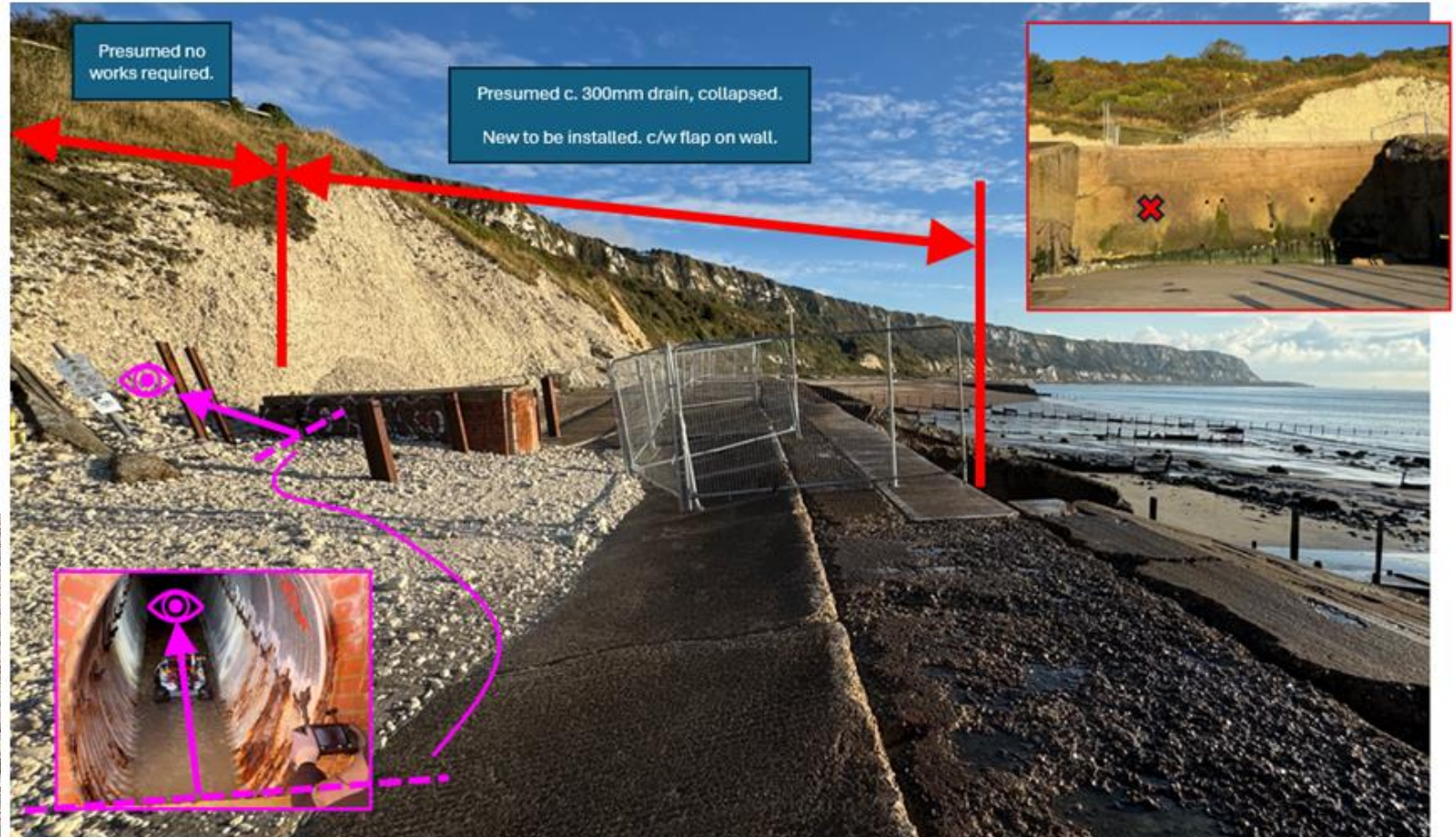
Figure 12. Walkway Drainage Repair Extents – 01/11/2024
