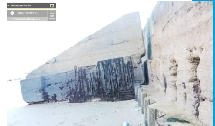
Figure 27. Bay 12 to 13 Buttress
