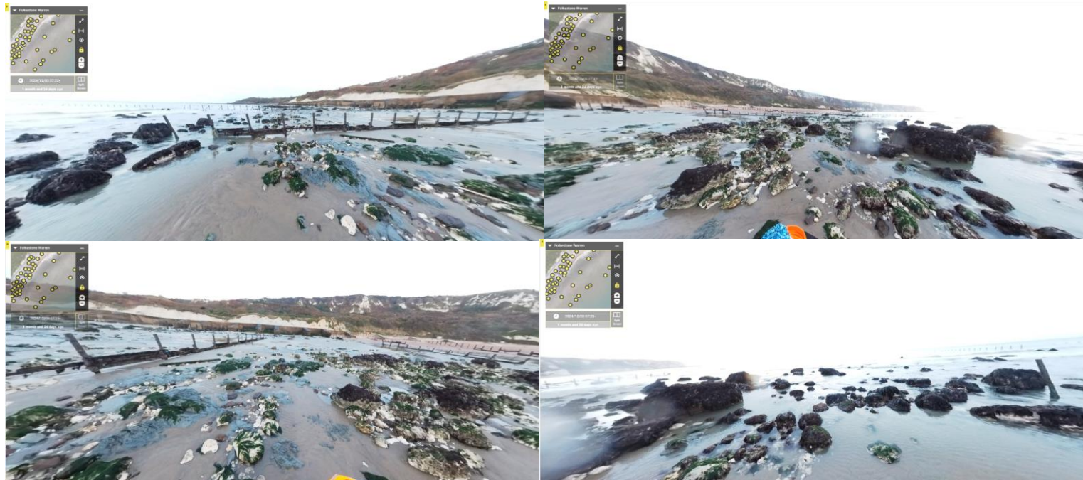
Figure 20. Holobuilder Scene 09 – Foreshore and Debris Extents adjacent to Bay 27 – Low Spring Tide
