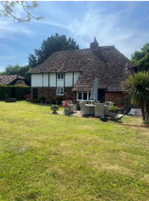
Rear of listed building – garage to be converted out of view.
