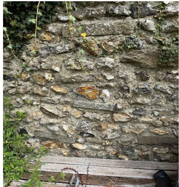
Correct finish of mortar (brushed).
