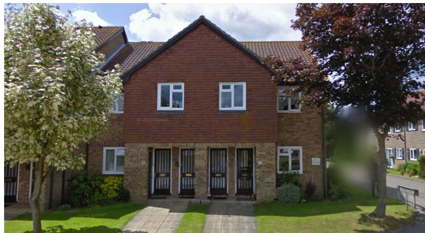
3 Station Road, yellow brick, clay hanging tile, plain roof tile
