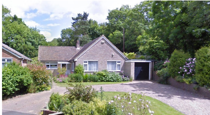
1 Greenbanks - Single-storey, brick, pitched roof
