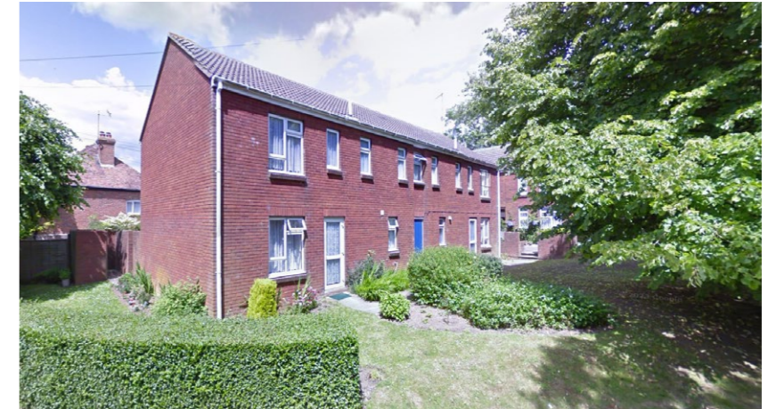
4 Greenbanks - two-storey, red brick, plain roof tile
