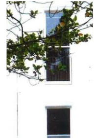
railings in upper window
