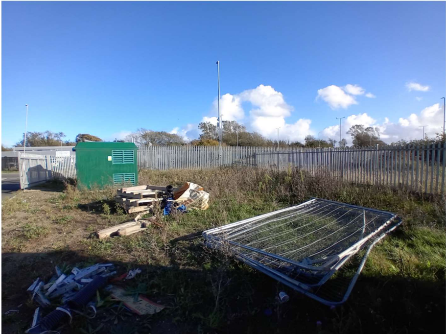
Photo 3: Site interior, facing east
