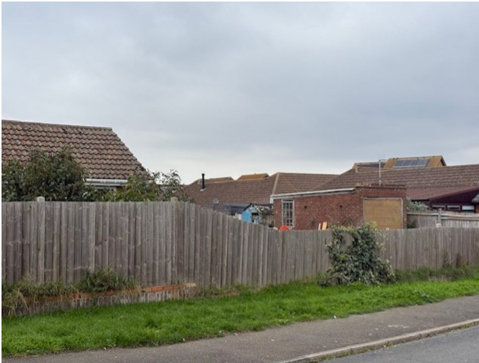
Figure 3: Site Photo looking towards the garage which is to be replaced and relationship with neighbouring property
