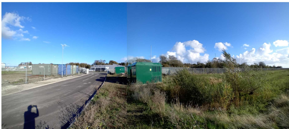
Photo 5: Site, facing east (substations not within red line)
