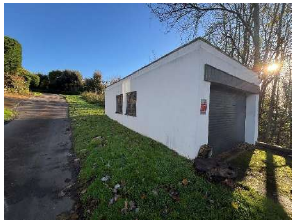
Photo 1: Garage building (B1), with 'Negligible' suitability to support roosting bats.
