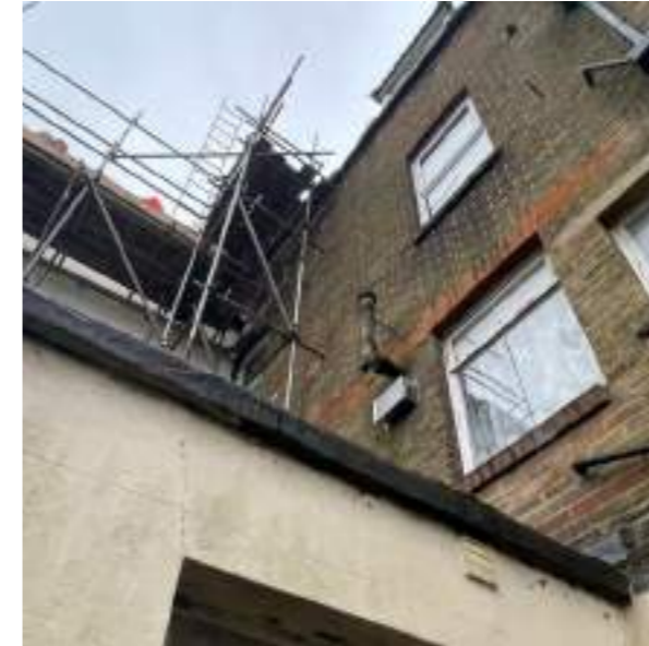
Existing flat roofing system
