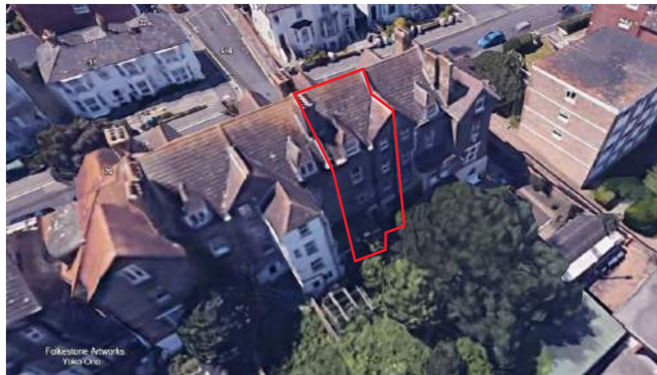
Aerial photo taken from Google Earth
