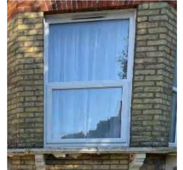
Existing UPVC windows
