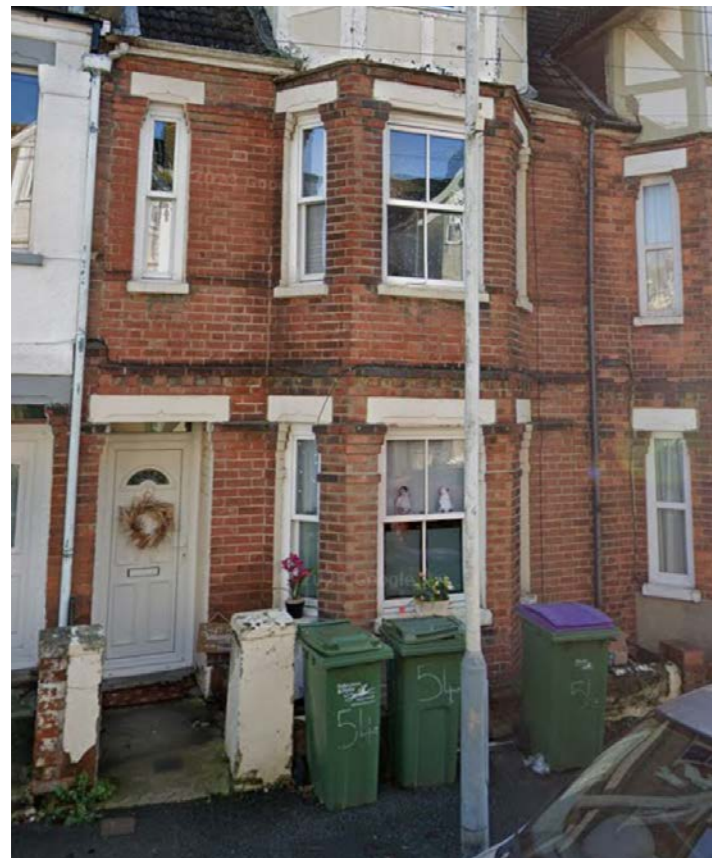
Image of existing bin location
