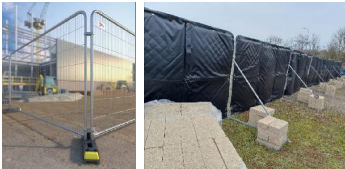
Figure 6: Example of HERAS fence panels and installation of fencing on site.
