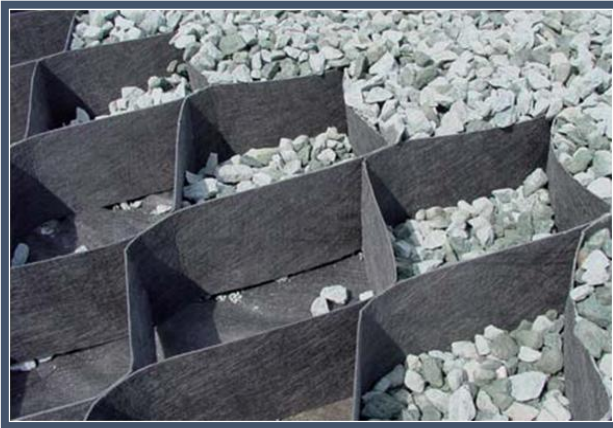
Figure 11 Examples of Cellweb filling with angular stone
