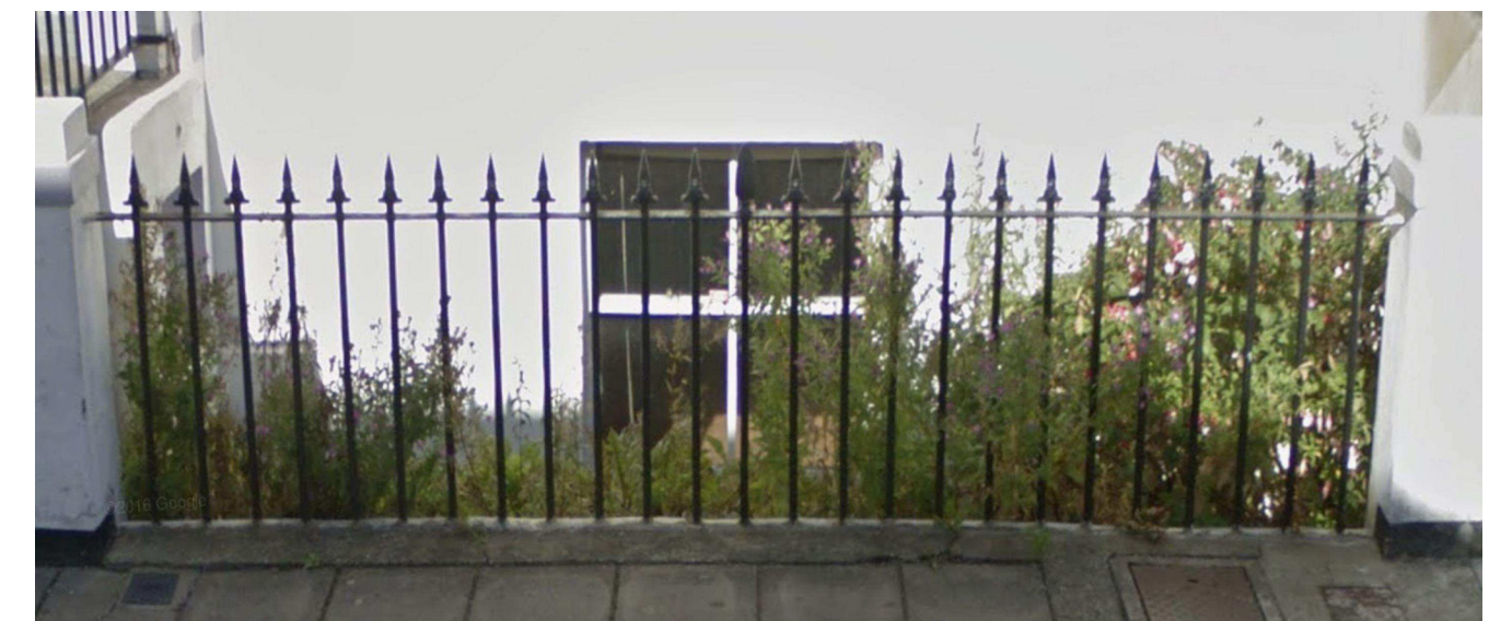
Photo of existing wrought iron railings to be replicated
