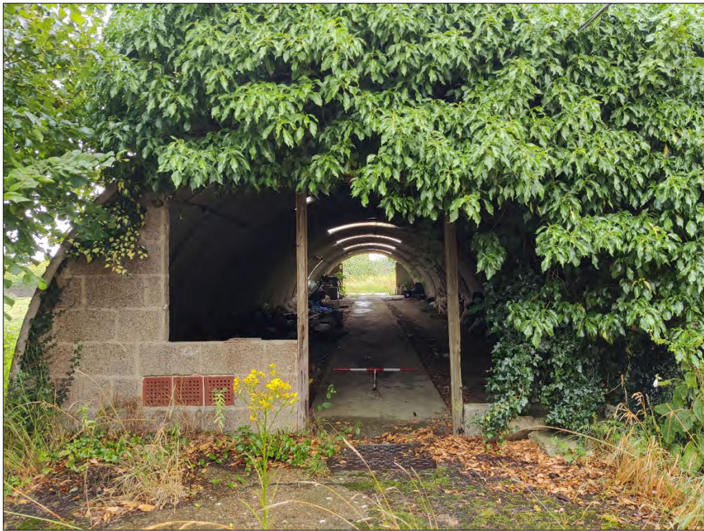
Plate 4: the Nissen Hut facing east.
