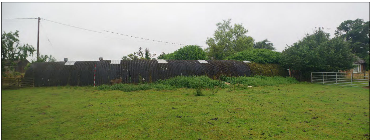
Plate 1: Nissen Hut facing south.
