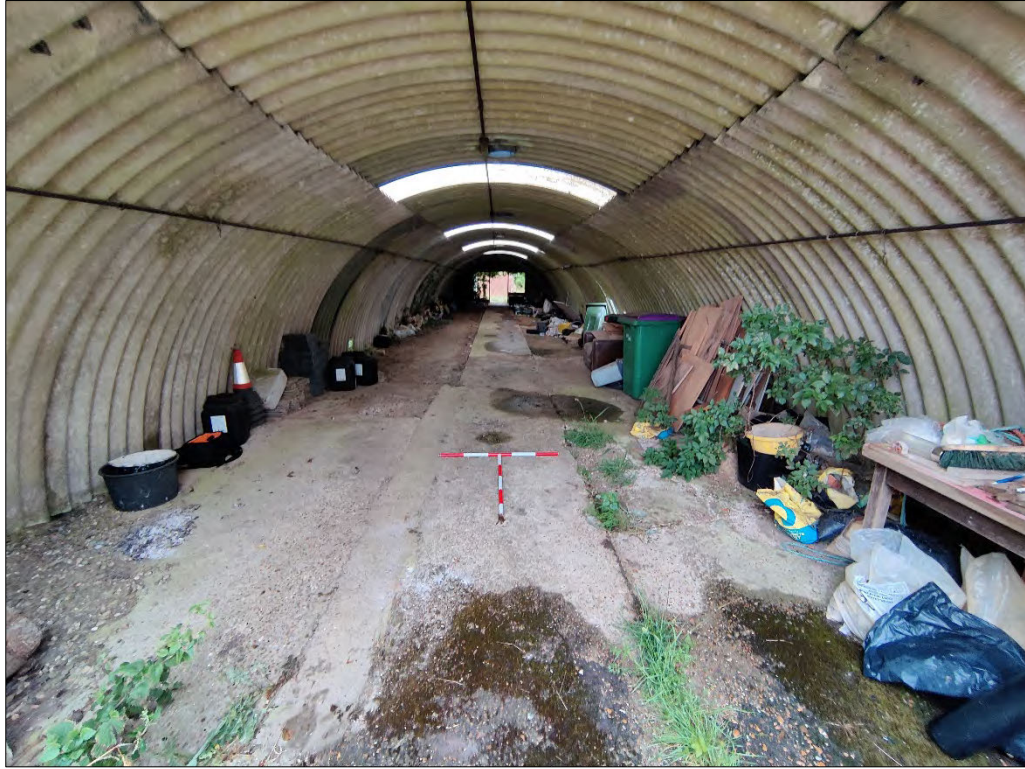
Plate 5: internal view of Nissen Hut, facing west.
