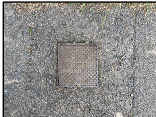
Plate 12. Small drain cover immediately adjacent to short track providing access to Site.
