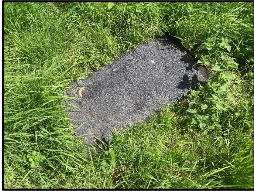
Plate 15. Several rubber mats noted along the edge of the Site boundary.
